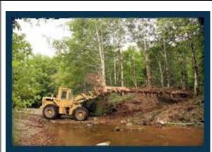
**Figure 17. Moving large woody** debris into the stream channel to re-establish structure in a 1-mile stretch of Sal Creek
